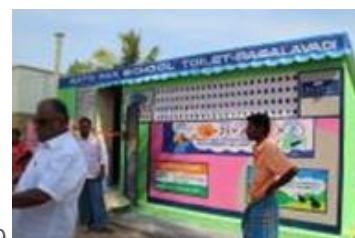
SATO toilet installed for Pagalavadi School in Trichy, India
