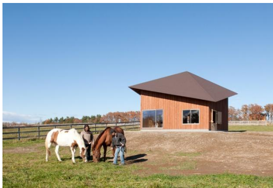
Top Prize of the 2nd Competition Keio University (Japan) / BARN HOUSE Completion: November, 2012 Photo by Shinkenchiku-sha.
