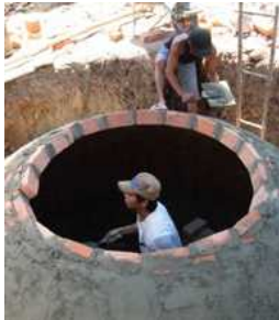
(Upper left) Top part of fermenter (Lower left) Fermenter is large enough for an adult to get in (Picture taken in the construction period)
