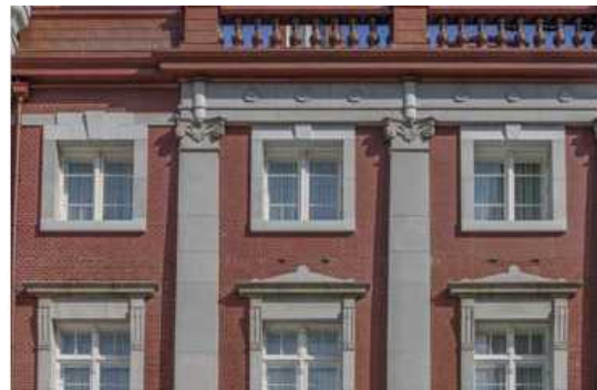
▲ Face bricks re-creating color variation (3rd floor part)
