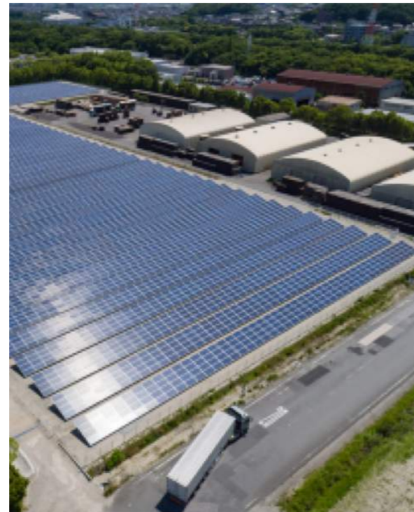
LIXIL CHITA SOLAR POWER (Generated energy in FYE2018: approximately 6,300MWh)
