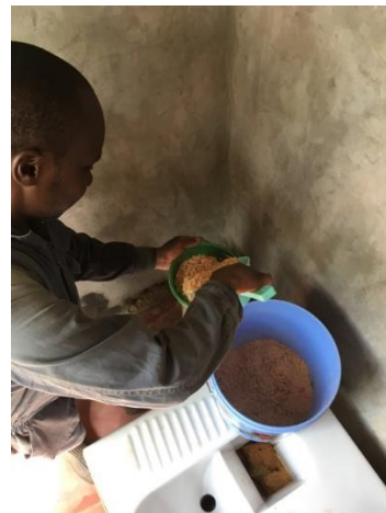
The Green Toilet System separates liquid and solid waste to prepare it for safe treatment and conversion into fertilizer for crops. Solid waste is treated using an aerobic composting technology, while liquid waste is treated using a method developed by an environmental organization in Japan, BMW Technology Association Inc.
